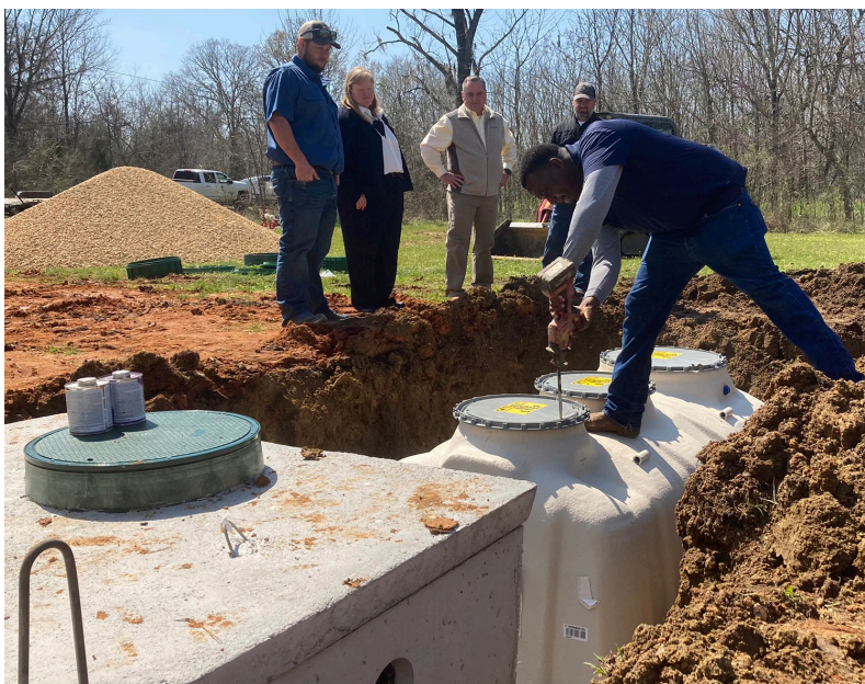
Septic Tank Installation
